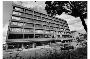
Murtenstrasse 24 (under construction)
